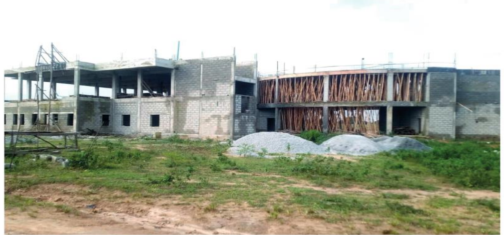
Frontal view of ICT Centre.
